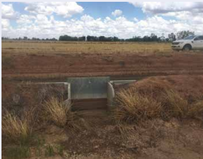
IMAGE 2: Old school slide gates used in manual irrigation.
